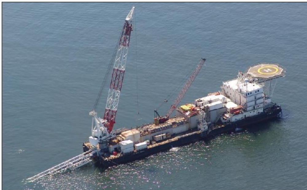
Figure 3-5 Example of pipelaying vessel (nearshore)
