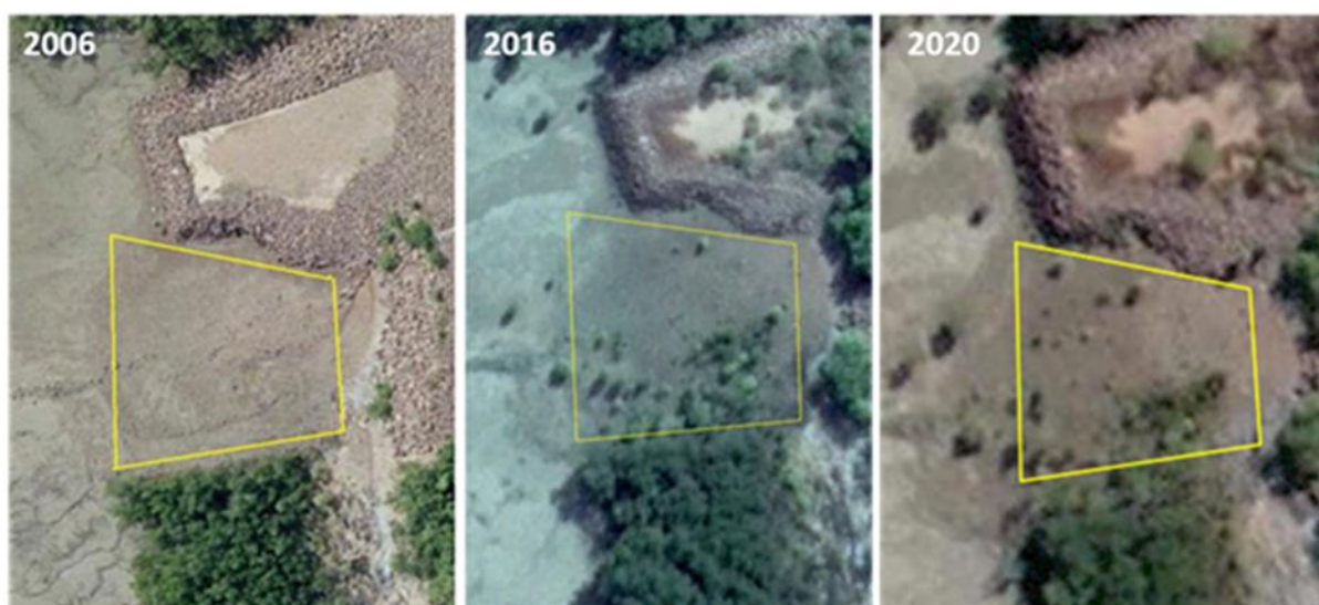
Figure 7-6 Aerial photographs of the pipeline shore crossing shortly after construction in 2006 (L) a decade later in 2016 (centre) and in 2020 (R).
