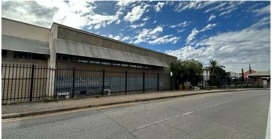
Figure 19 – Fenced off SAPOL building compound from Gaol Road
