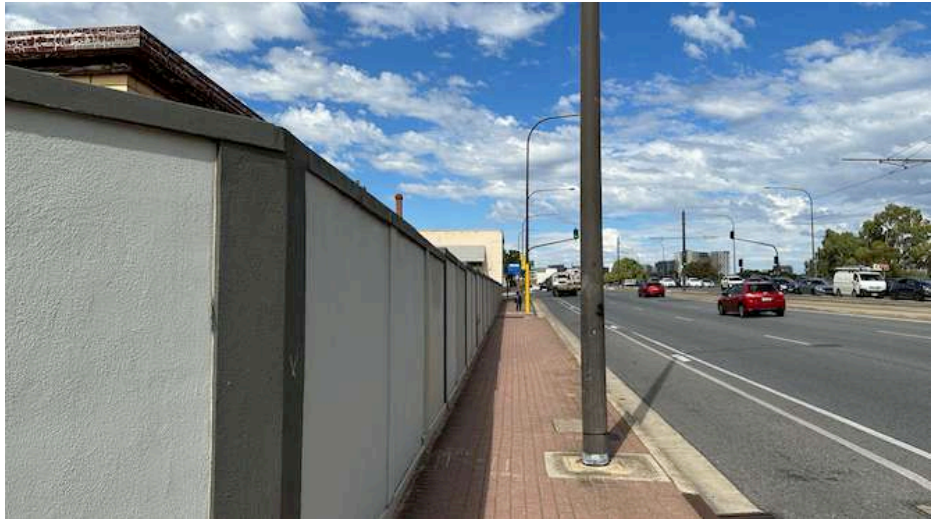
Figure 36 – Port Road (within Park Lands) interface with SAPOL site
