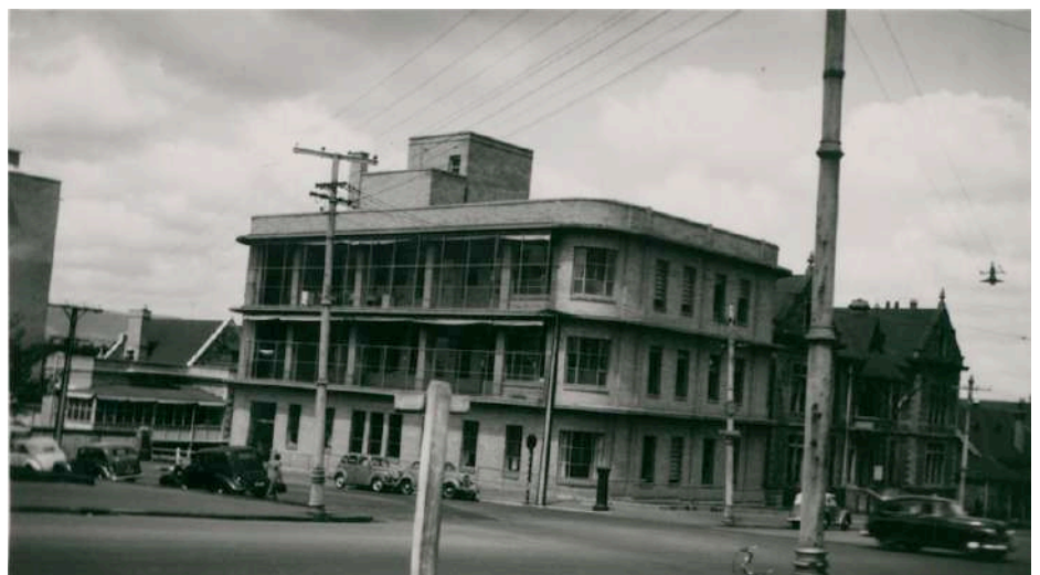
Figure 55 – Mitchell Building at the Adelaide Children's Hospital, 1952 [Source: SLISA, Image No. B_12324]
