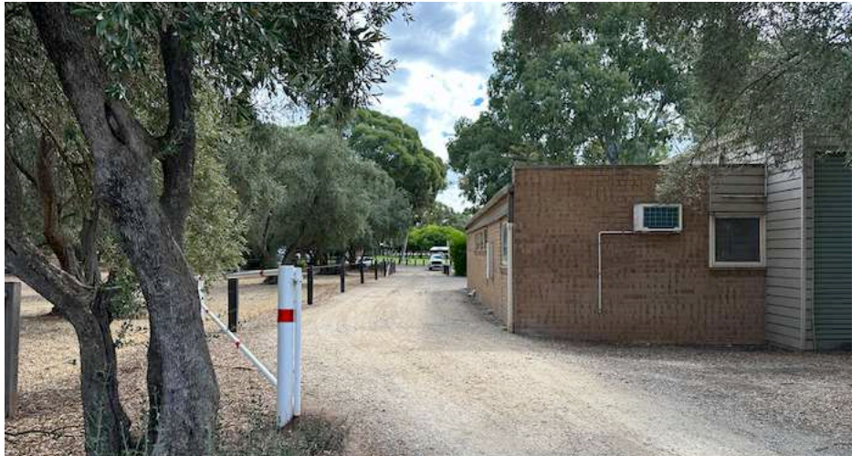
Figure 27 – Adelaide City Council maintenance facility to the north of Kate Cocks Olive Grove
