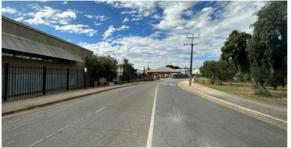
Figure 18 – Gaol Road looking north, with SAPOL building compound to the left and fenced off former agistment to the right
