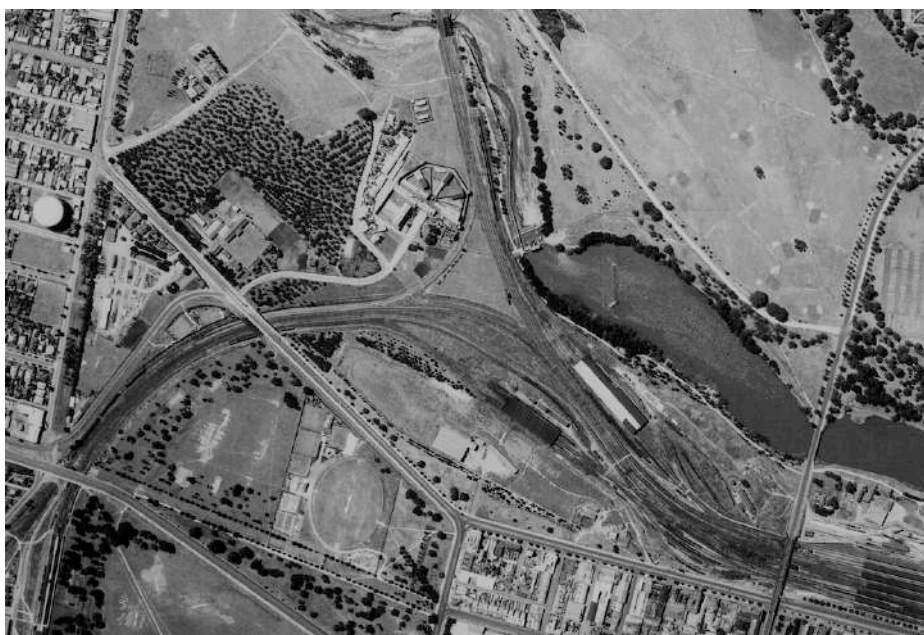
Figure 66 – Aerial photograph, November 1935 [Source: Geosciences Australia]
